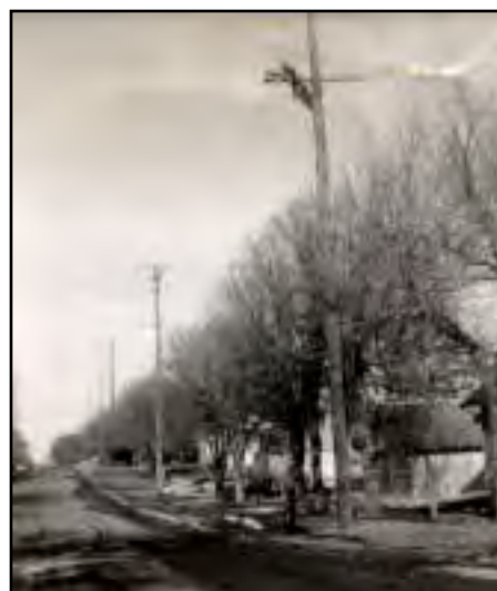
This last picture is in Creighton where there was an inverted crossing. Our toll line was above the secondary power. I believe we were about 45 feet up.
